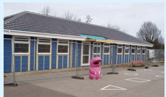
The Nurture building under construction
